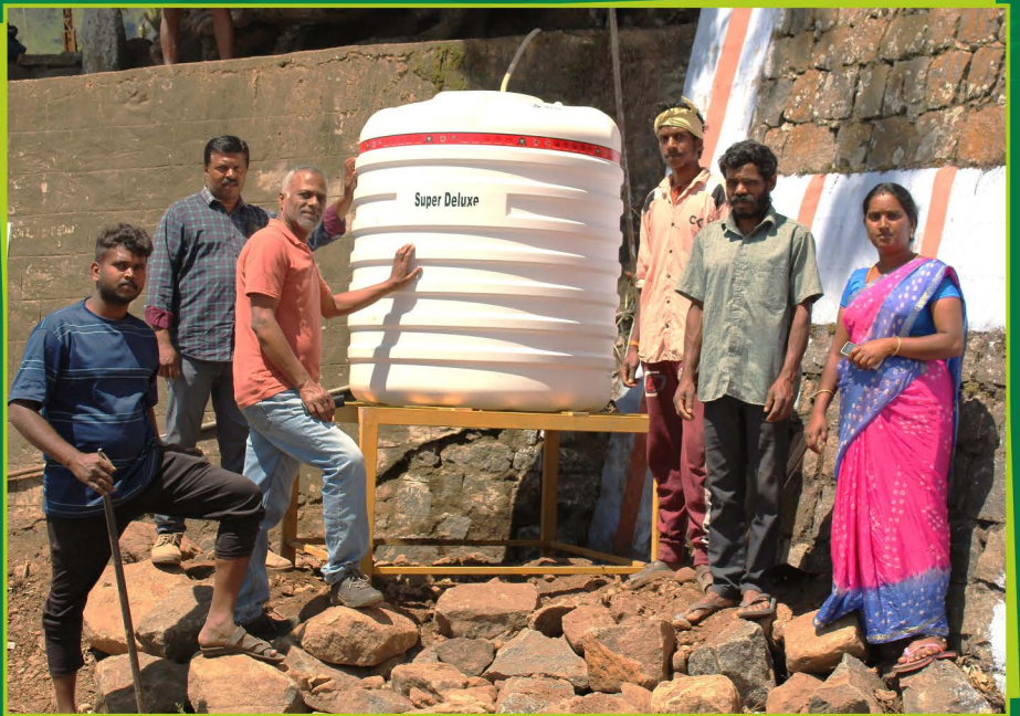
◆ New Community Water Tank
