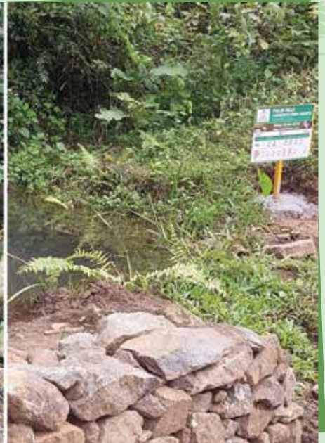
◆ Restored Spring w Testing Results
